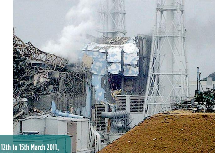
the fuel began to melt, generating hydrogen which built up in the buildings housing the reactors. Explosions blew out the superstructures, leading to fears of reactor containment cracking.
